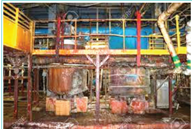
Figure 1: Badly installed and maintained refrigeration plant
